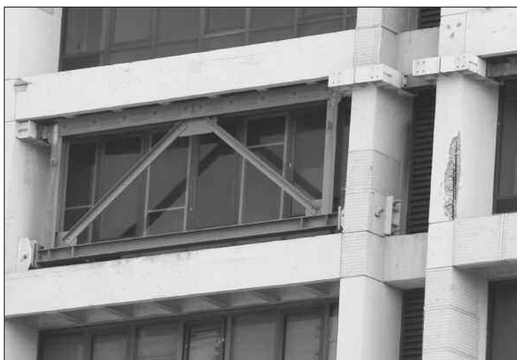
At right, rusting reinforcing rods force concrete to flake off. The braces, seen across the window, help hold the building up.
